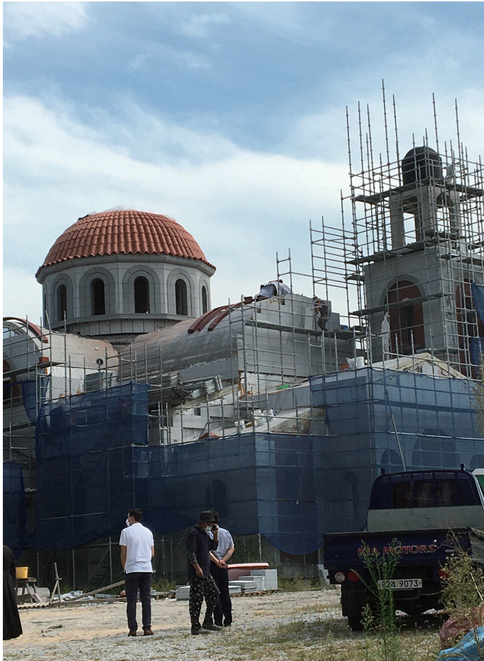
The Holy Church of the Assumption under construction of the Virgin in the city of Jeonju.
